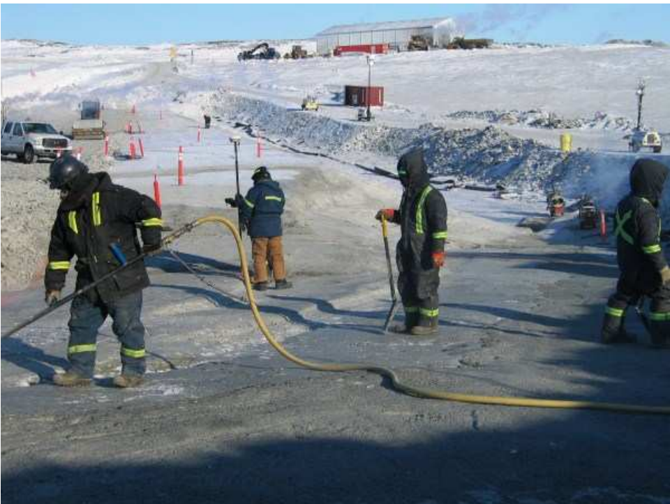
Photo 5: Preparing surfaces with compressed air.
