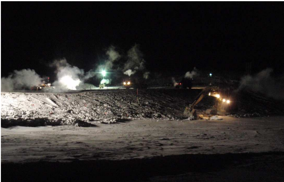
Photo 17: 330 Excavator placing ROA and shaping 4H:1V downstream slope.
