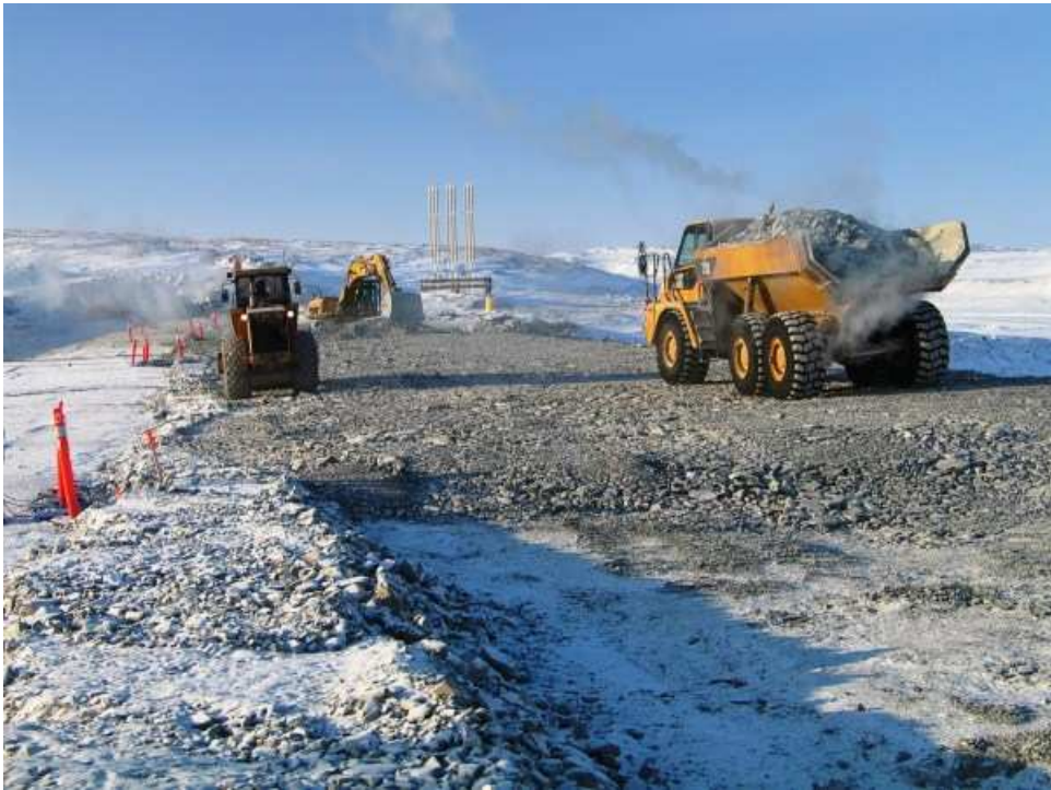
Photo 10: Placing ROQ on downstream side.
