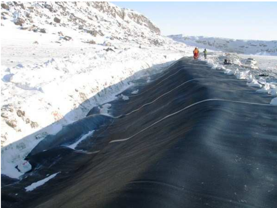
Photo 12: HDPE . Layfield in the background welding seams.
