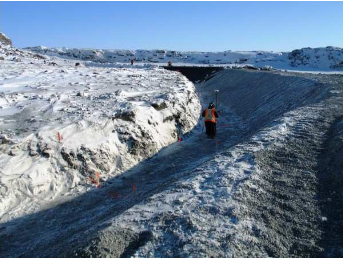
Photo 14: Surveying. Setting grades for bentonite
