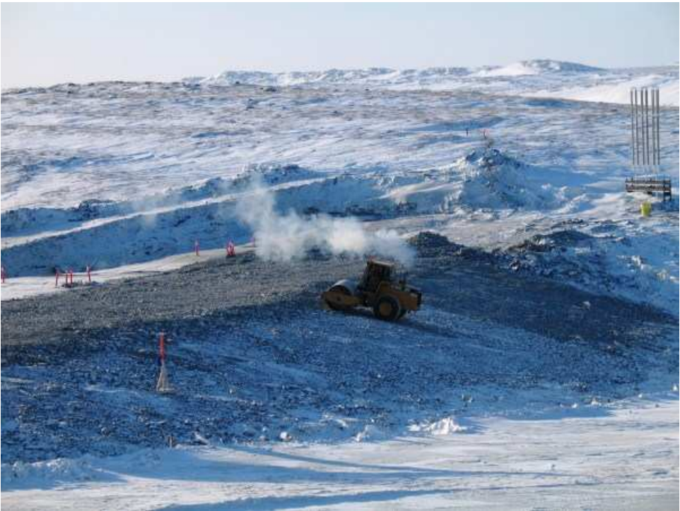
Photo 11: 10 ton packer working on sideslopes
