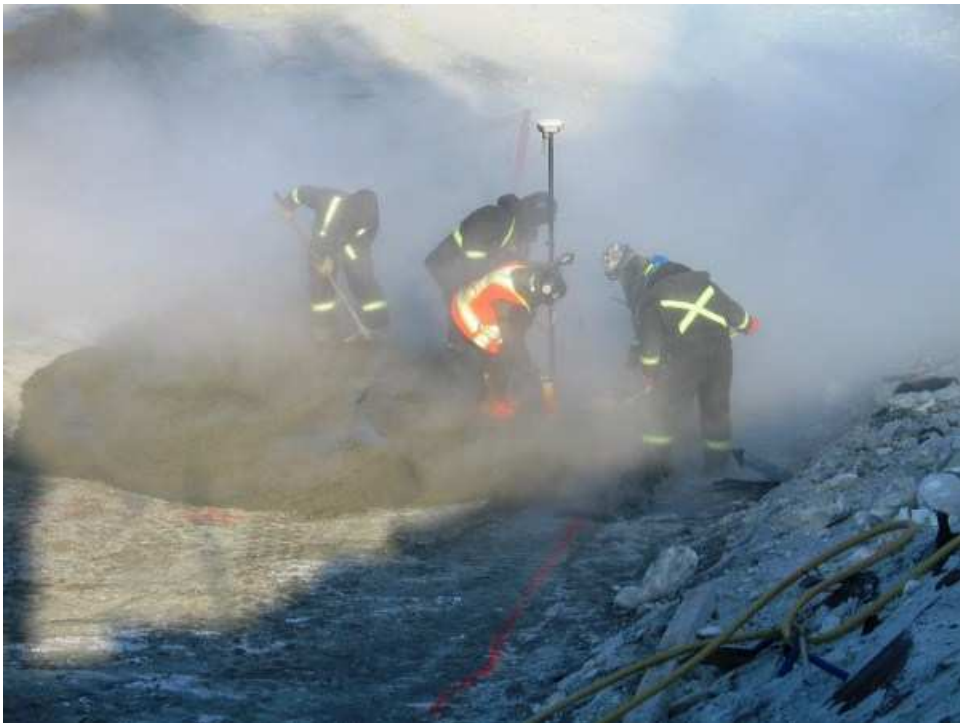
Photo 6: Survey control; workers raking slope. Steam on a very cold day
