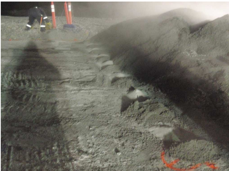
Photo 16: Multi bead thermistor strings installed at station 1+30 at elevation 33.5m today.
